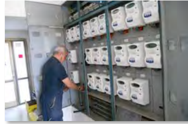
Basements and sewages
